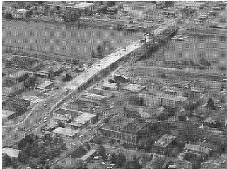
New Allen Street Bridge.
