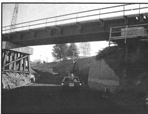
Then: Widening Wine Country Road and increasing height under the railroad bridge.
