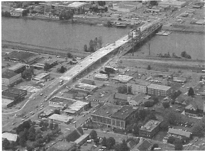
New Allen Street Bridge.
